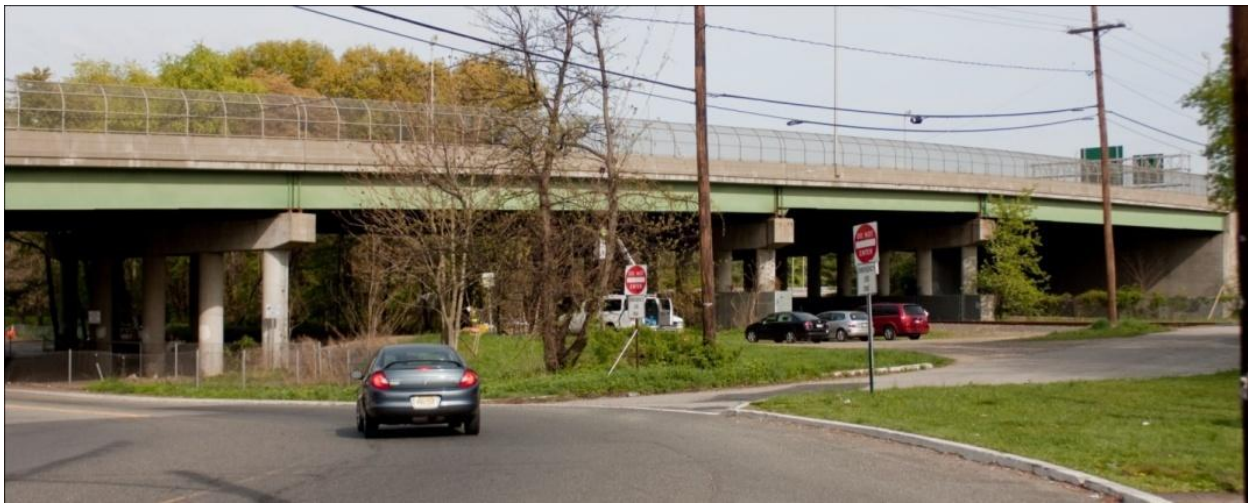
Figure 1. US 202/NJ 23 Bridge used in International Bridge Study
