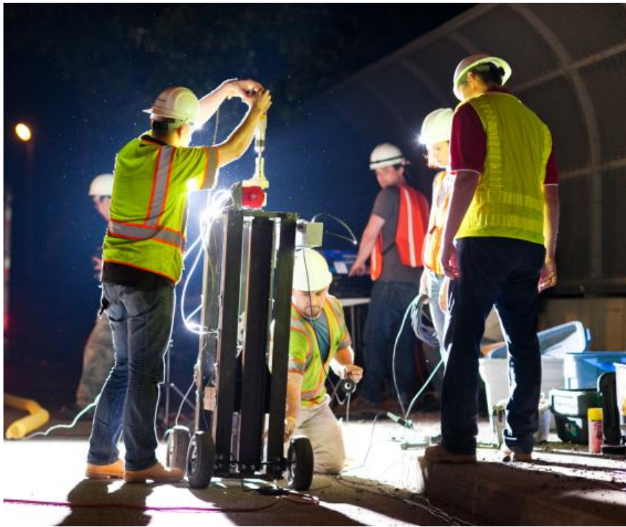
Figure 4. Automated drop hammer system with rebound control designed by Drexel team
